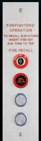
(F) INTERMEDIATE HALL STATION WITH FIRE SERVICE DEVICES
